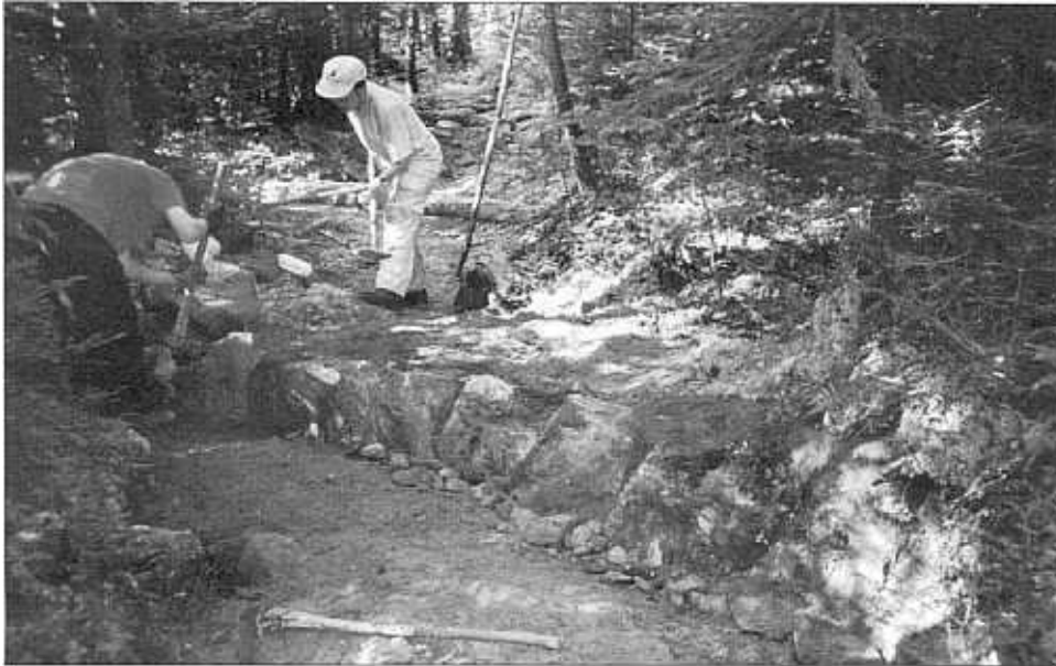
One of many new rock water bars on the Kate Sleeper Trail, built during a mid-summer trip with scouts from Marion, MA.
