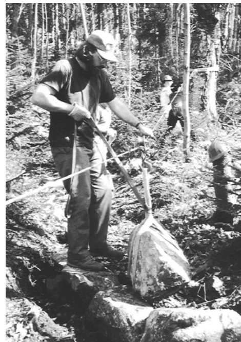
A few years back on Lawrence Trail: Chris guides a rock for a new waterbar while Judy and the griphoist do the heavy lifting. Photo: P. Smart
