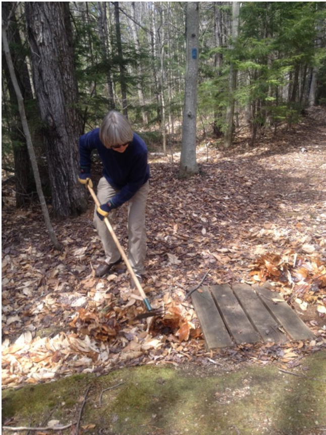
Chele clears a water bar on the Cabin. Photo by Helen Steele.
